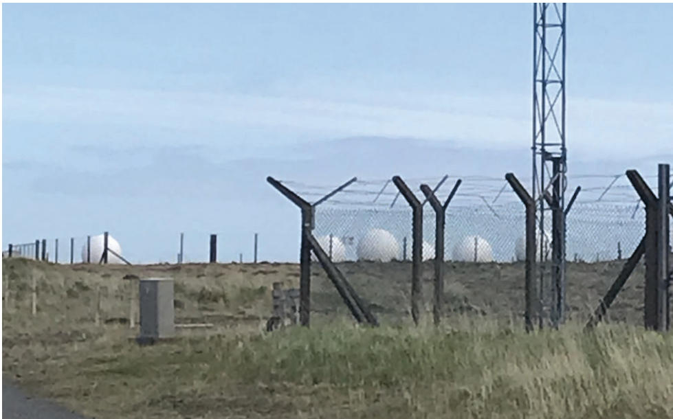
Radomes at Baltasound Airport
